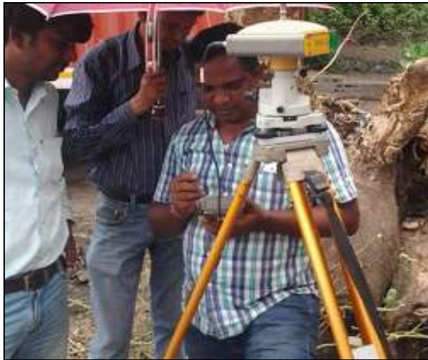
Survey Work for Construction of Garden Reach Flyover Kolkata
